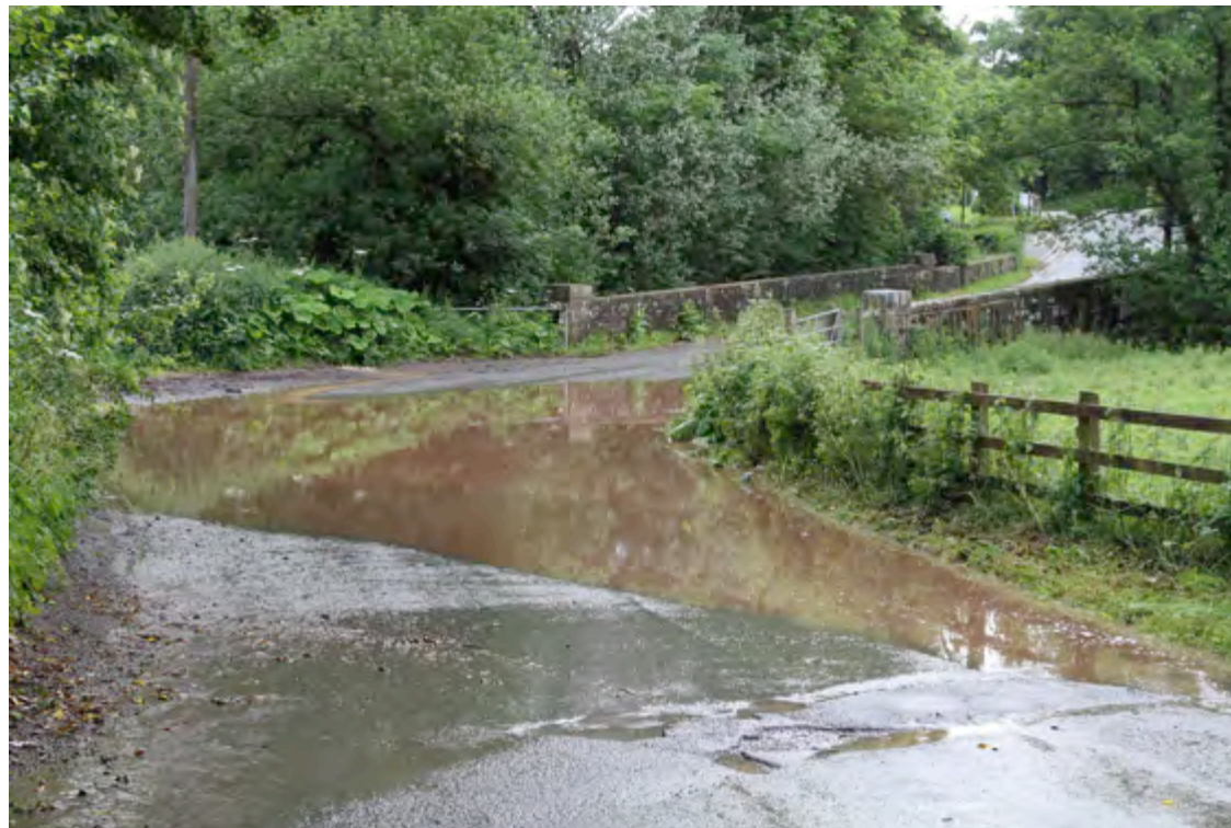
Flooding at entrance to the village from the A44
