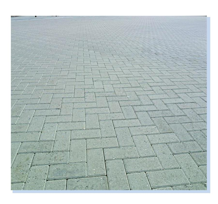
Concrete block paving 'natural' to match existing footways
