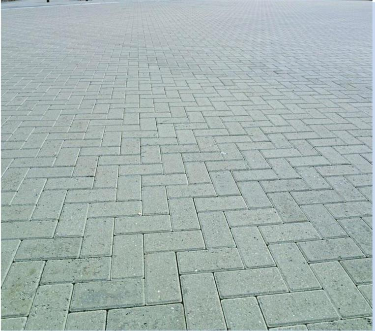
Concrete block paving 'natural' to match existing footways
