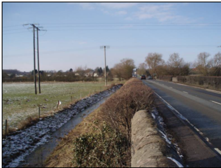
Fig A6.15 Relief culvert at A465 Aylestone Hill
