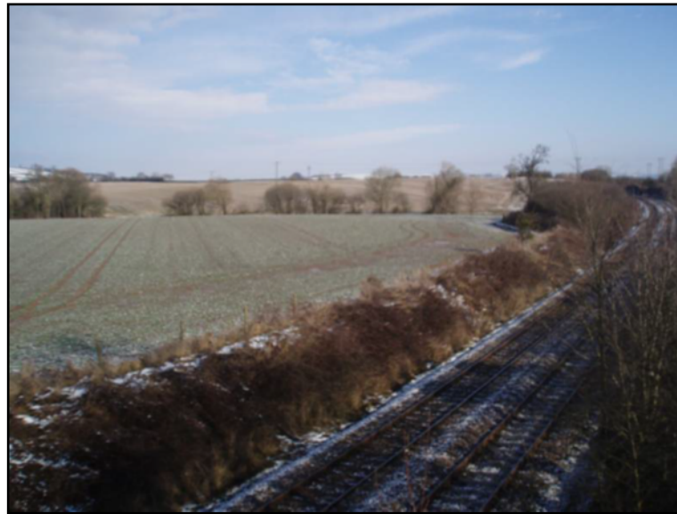
Fig A6.12 West side of existing railway line north of A4103 Roman Road
