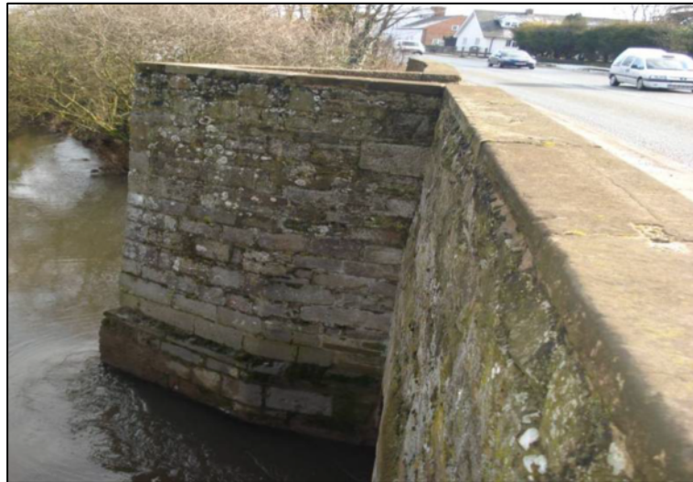
Fig A8.5 The Lugg Bridge (Cutwaters on northern side)
