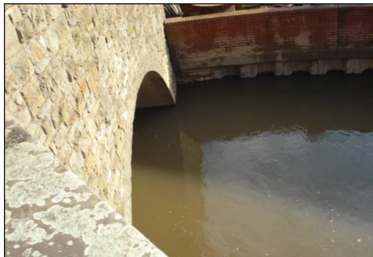
Fig A8.4 The Lugg Bridge masonry arch
