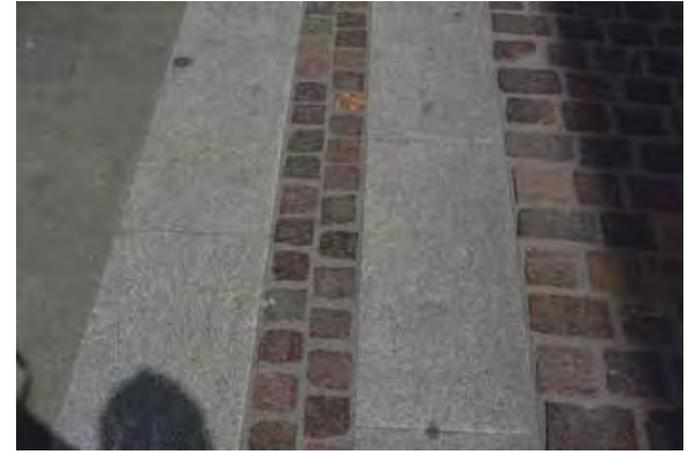
Granite kerb and Porphyry setts, kerbs to be laid flush with paving
