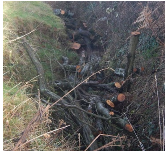
Figure 9.11 Natural in-ditch seepage barrier – Herefordshire Council (2020)
