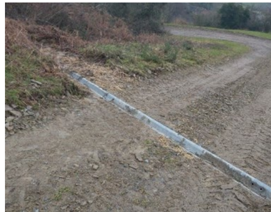
Figure 2 Cross drain – NFM Construction grant recipient (2021)
