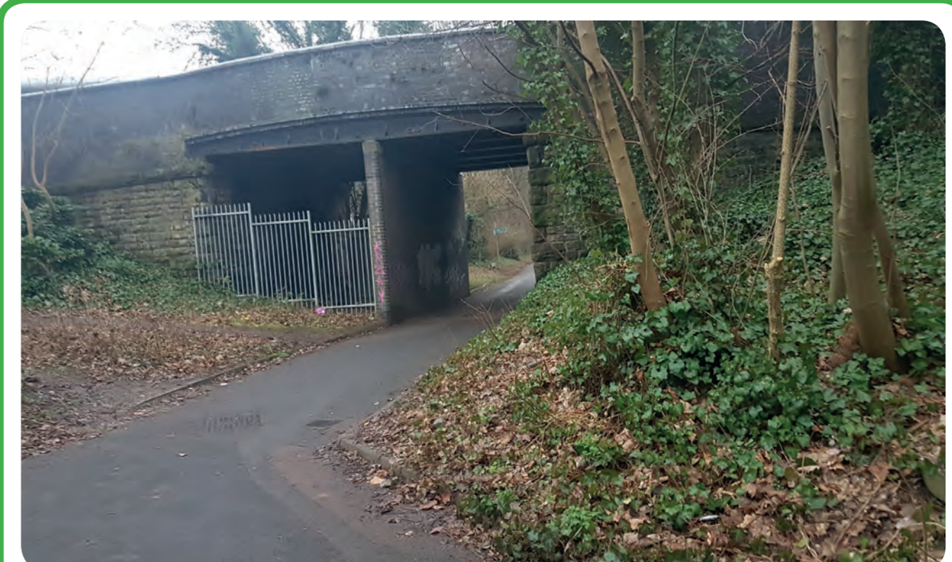
Lighting improvements on Great Western Way under bridge
