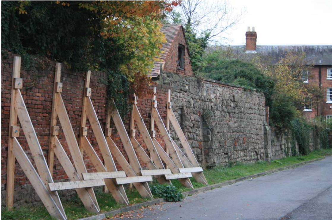
The failed brickwork stretch of wall immediately north of the Black Lion plot, prior to repairs
