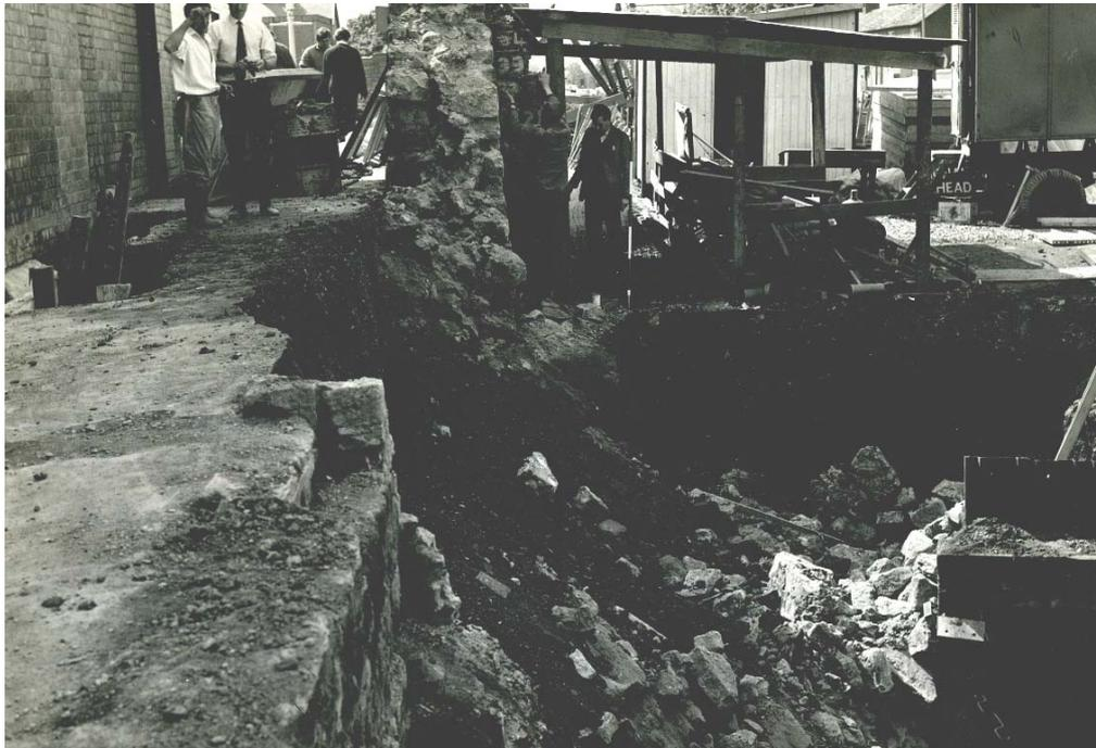
The north end of the Gunners Lane wall in 1968 following the collapse of masonry into the underpass excavations alongside (Contract photographs file, Hereford City Council)
