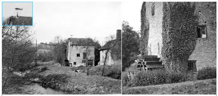
Two photos of Aymestrey Mill taken during the 1950s, well after it became disused, note the bridge over the 'tail leat' and the fishy weather vane! Now a listed building.
