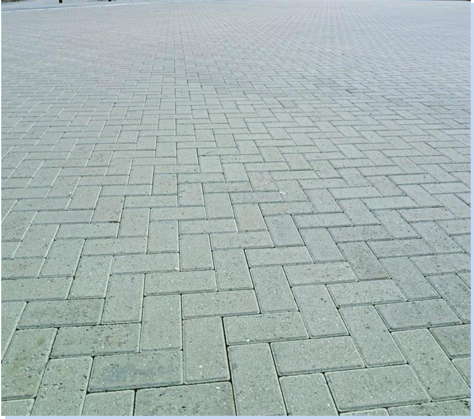
Concrete block paving 'natural' to match existing footways
