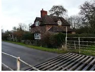
Lodge at East entrance to Homend Park looking east from G, Map 10
