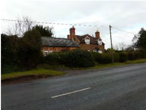
House at Lower Eggleton on North side of A4103 looking from E, Map 10
