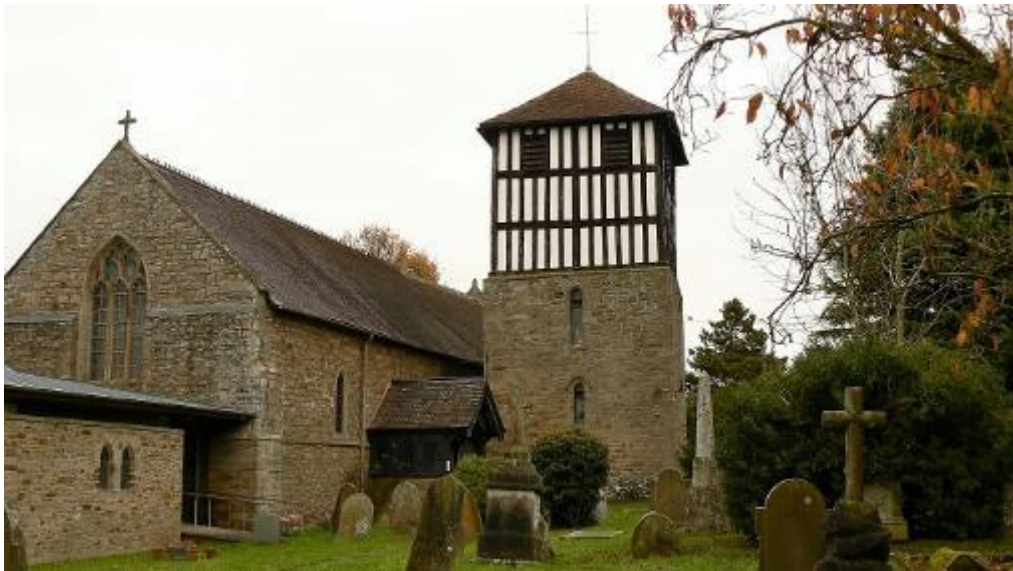
viii St Bartholomew's Parish Church, one of the area's limited community facilities
