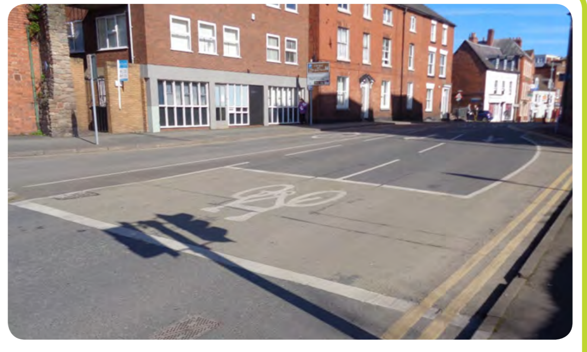
Existing advanced stop line on St Nicholas Street at junction with A49 to be replicated on all arms
