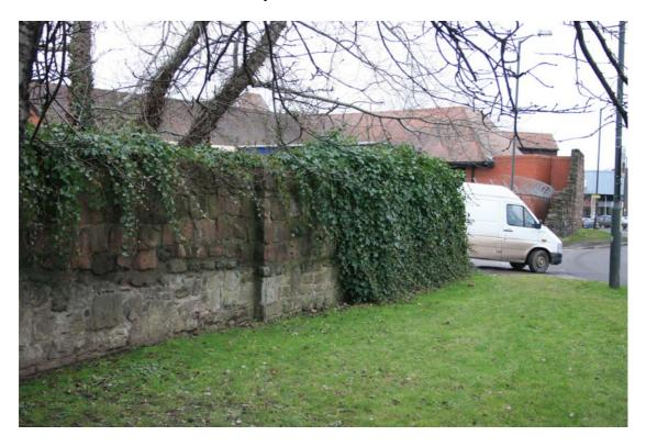
Looking west towards the north-east end of the section 7 (c.1983) wall beyond the Tesco vehicle exit. The section 8 wall in the foreground consists of base courses surviving from the 1968 wall raised by the addition of the distinctive red c.1983 Tesco-Shoesmith masonry
