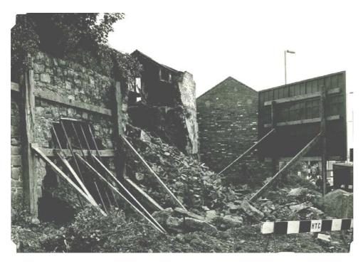
The south end of section 3 looking south. Photograph of September 1968 showing collapses immediately north of the electricity sub-station (Hereford City Council contract photographs file)
