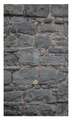
Detail of the suggested 'primary' build character masonry, seen in section 1 and elsewhere, consisting of large square blocks with short, intermittent levelling-up courses
