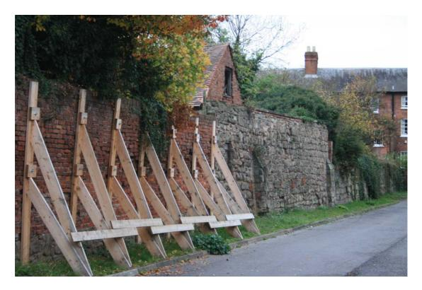
The failed brickwork stretch of wall immediately north of the Black Lion plot, prior to repairs
