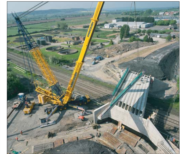
We will continue to update and improve the transport asset
