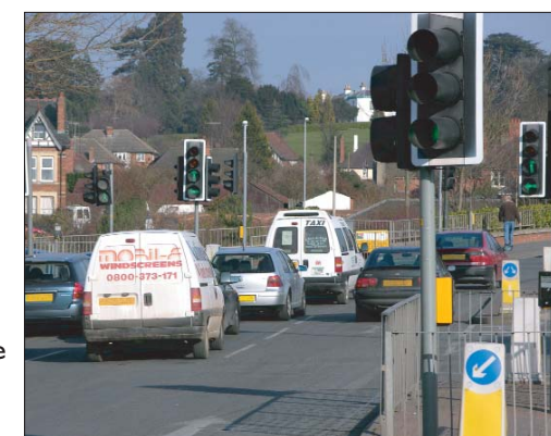
6 monthly checks of all signal equipment and the ability to react quickly to any loss of service ensures traffic flow is maintained
