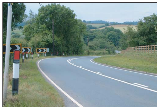
Combined improvement schemes provide a complete treatment
