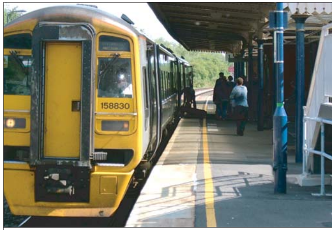
Leominster Rail Station
