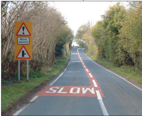
Signing and marking scheme using a red central strip to guide drivers through the hazard
